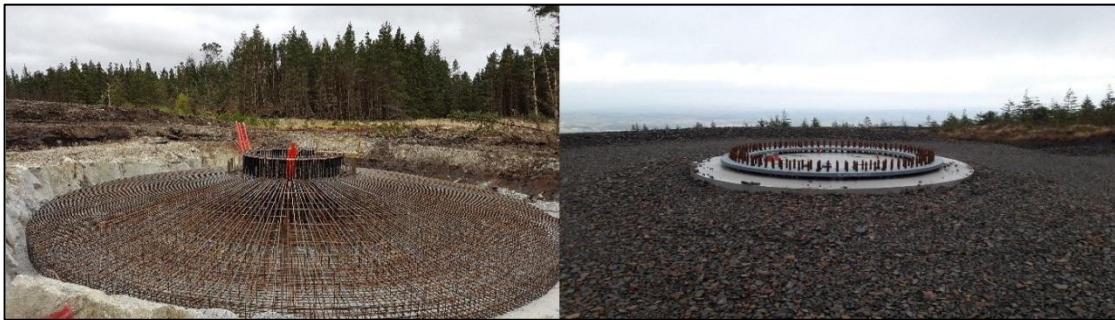
Plate 3-2: Turbine 'Anchor Cage' and finished turbine base
