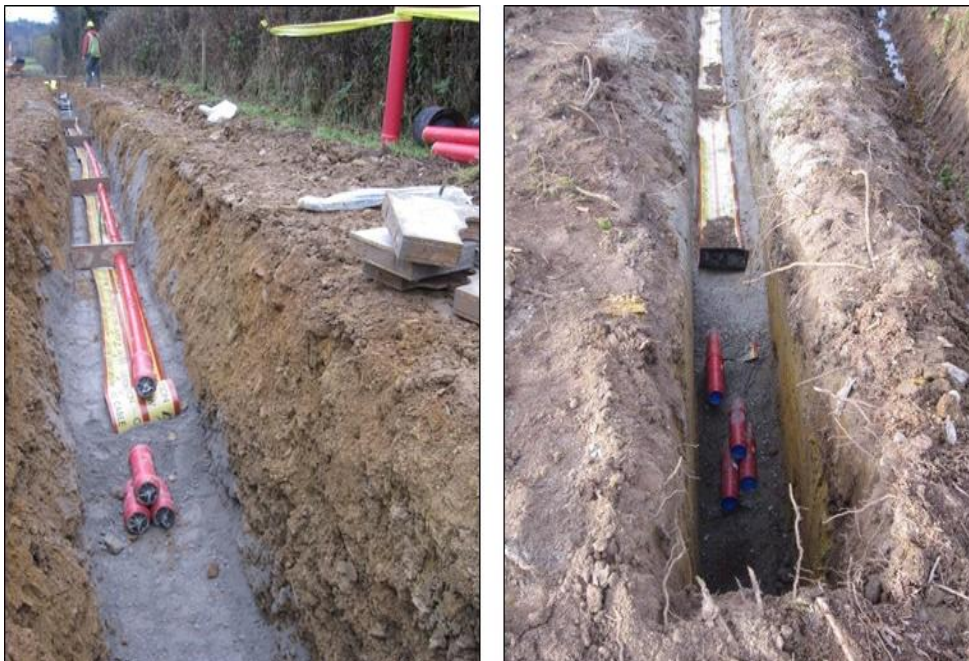
Plate 3-4: Typical Cable Trench View
