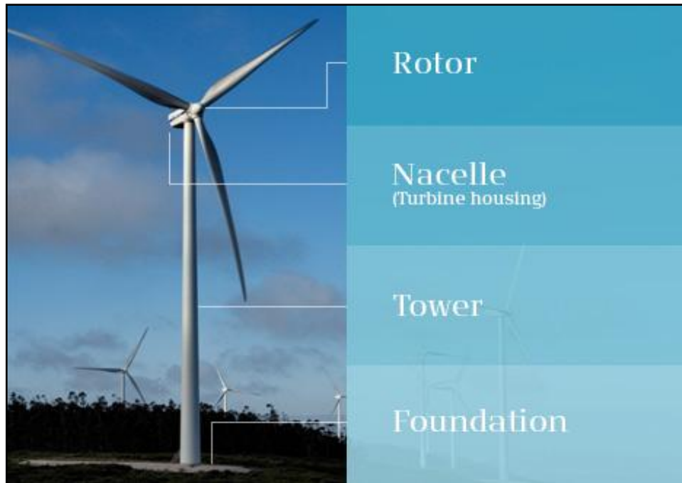
Plate 3-1 Wind turbine components
