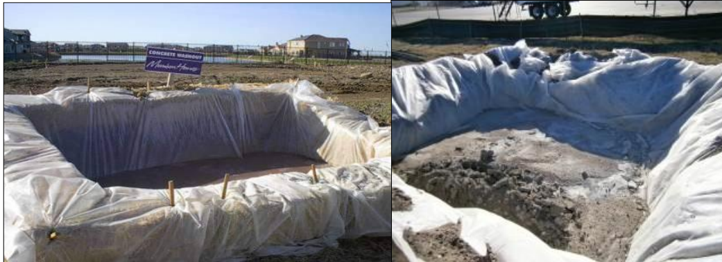
Plate 3-3: Concrete washout area
